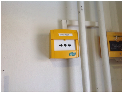
Air-conditioning emergency stop button
