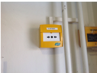
Air-conditioning emergency stop button
