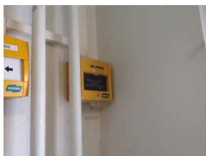
Smoke extraction activation button
