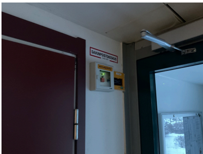
I-V emergency stop and smoke evacuation triggering
