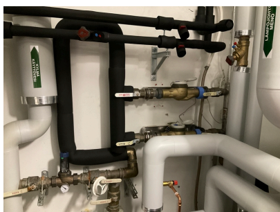
Water inlet shut-off
