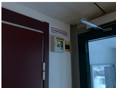
I-V emergency stop and smoke evacuation triggering
