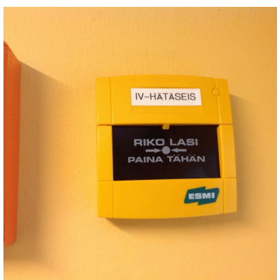
Air-conditioning emergency stop button
