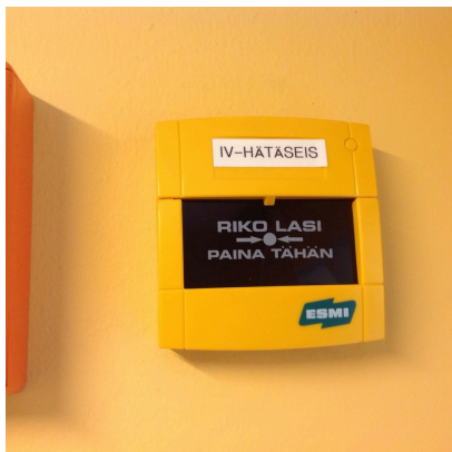
Air-conditioning emergency stop button
