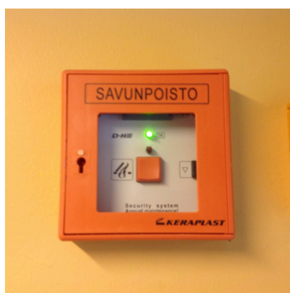
Smoke extraction activation button
