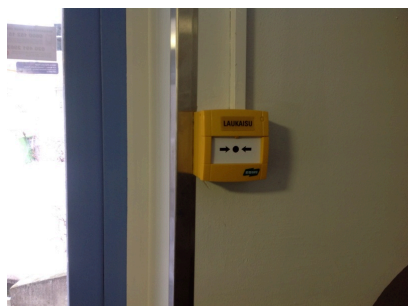
Air-conditioning emergency stop button
