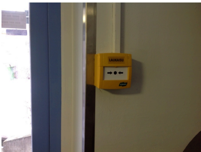
Air-conditioning emergency stop button
