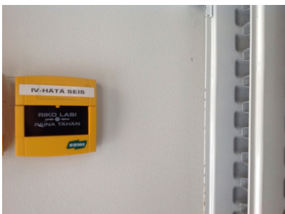
Air-conditioning emergency stop button
