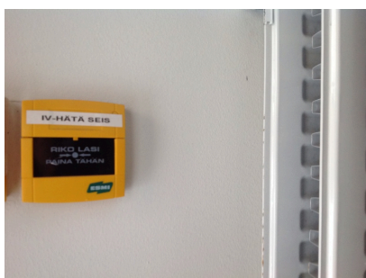
Air-conditioning emergency stop button
