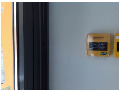
Smoke extraction activation button
