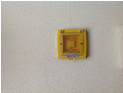
Air-conditioning emergency stop button
