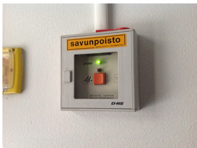
Smoke extraction activation button
