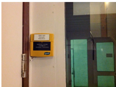
Air-conditioning emergency stop button
