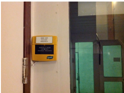
Air-conditioning emergency stop button
