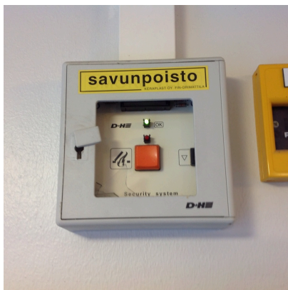
Smoke extraction activation button
