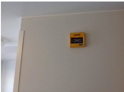
Air-conditioning emergency stop button
