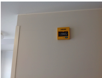
Air-conditioning emergency stop button
