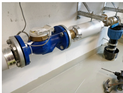
Main water seal in the heat exchange plant room
