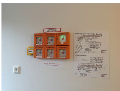
Ventilation system emergency stop and smoke vent buttons
