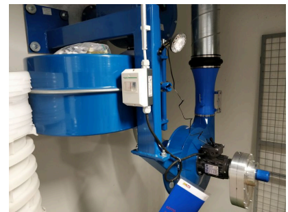
The air-conditioning equip- ment of the civil defence shel- ter
