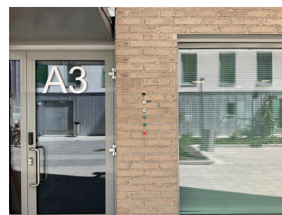
Standpipe locks next to the door to A3
