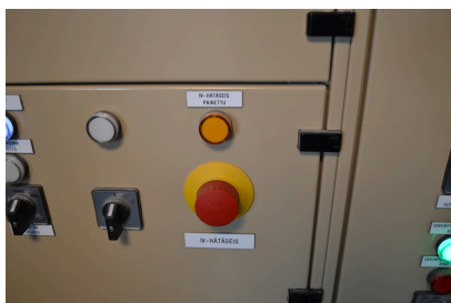
Air-conditioning emergency stop
