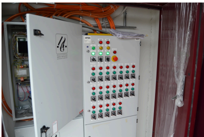
Smoke extraction activation panel
