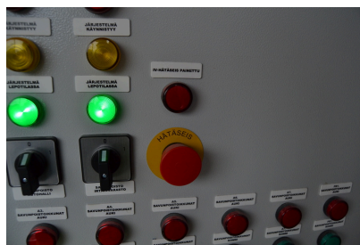
Ventilation emergency stop at the smoke extraction system
