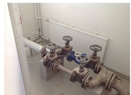
Main water stopcock in the bicycle store of staircase A
