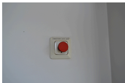
Air-conditioning emergency stop button
