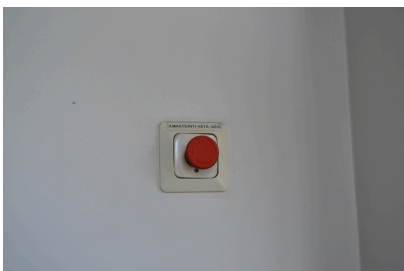
Air-conditioning emergency stop button
