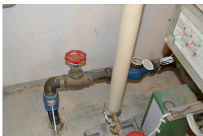
Main water cut-off valve
