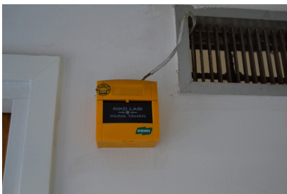
Air-conditioning emergency stop button
