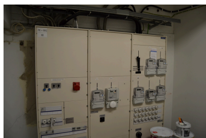
The apparatus of the main electrical switchboard
