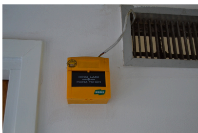
Air-conditioning emergency stop button
