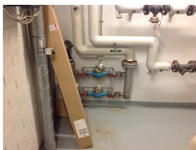
The main water cut-off valve in the heat distribution room
