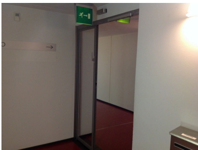
Automatically-closing fire doors in the floor corridors
