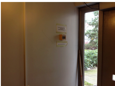
Air-conditioning emergency cut-off at the entrance of staircase B
