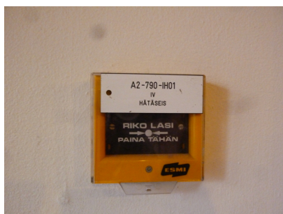
Air-conditioning emergency stop is located in the lobby of staircase A
