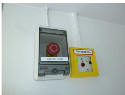
Air-conditioning emergency stop
