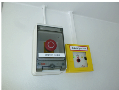
Air-conditioning emergency stop
