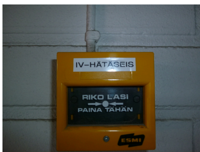
Air-conditioning emergency stop
