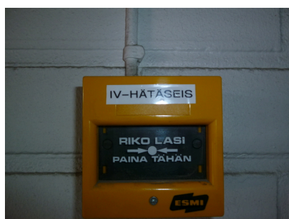
Air-conditioning emergency stop
