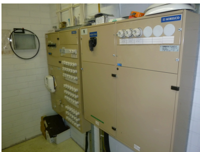
Electricity switchboard
