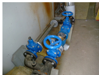
Main water stopcock, on the right side of the entrance of Tarmonkatu 6, staircase A
