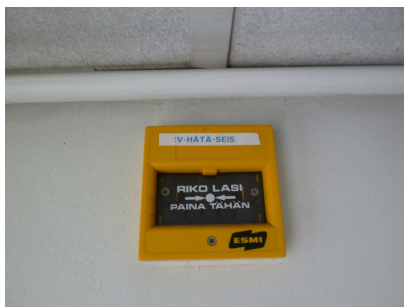
Air-conditioning emergency stop
