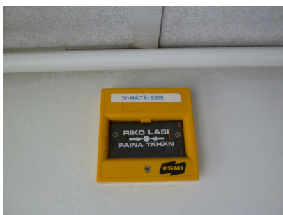
Air-conditioning emergency stop
