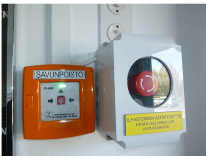
Air-conditioning emergency stop
