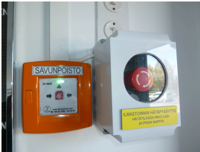
Air-conditioning emergency stop
