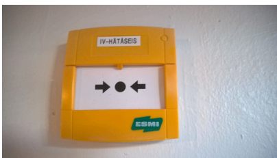
Air-conditioning emergency stop
