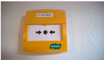
Air-conditioning emergency stop
