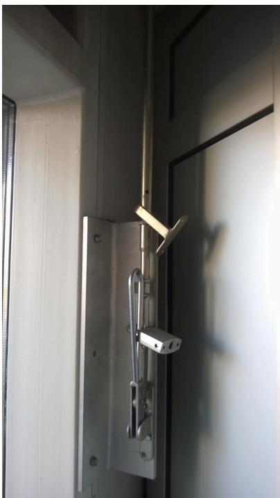
Manual smoke extraction activation
