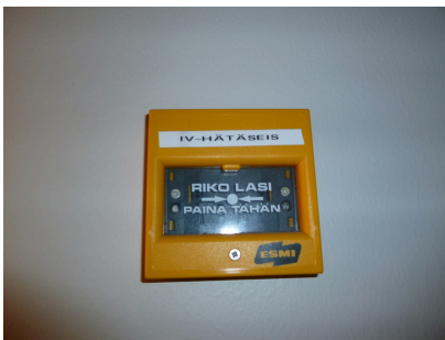
Air-conditioning emergency stop
