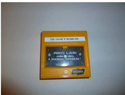
Air-conditioning emergency stop
