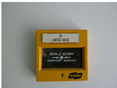
Air-conditioning emergency stop
