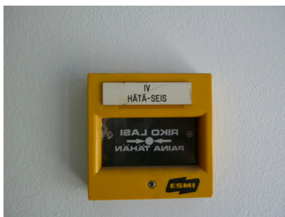
Air-conditioning emergency stop
