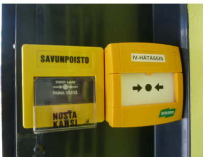
Air-conditioning emergency stop
