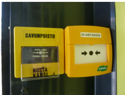
Air-conditioning emergency stop
