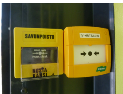
Manual smoke extraction activation
