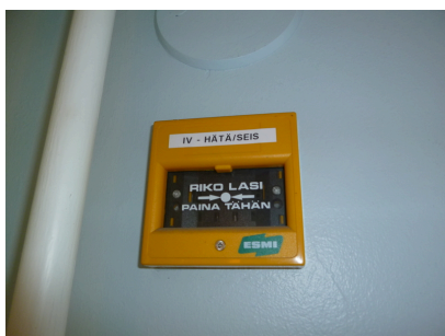
Air-conditioning emergency stop
