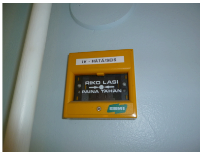
Air-conditioning emergency stop
