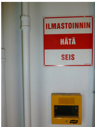
Air-conditioning emergency stop
