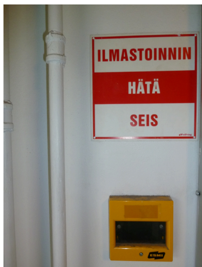
Air-conditioning emergency stop
