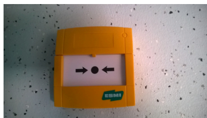
Air-conditioning emergency stop
