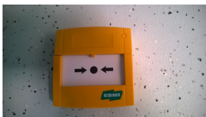
Air-conditioning emergency stop
