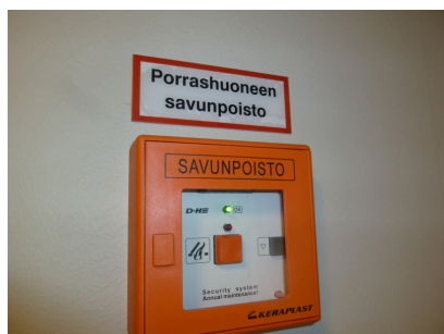
Manual smoke extraction activation
