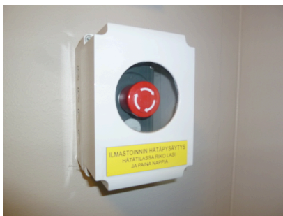
Air-conditioning emergency stop
