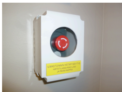
Air-conditioning emergency stop
