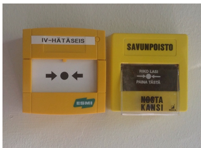
Smoke extraction activation button
