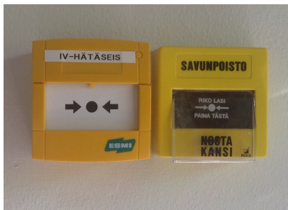
Air-conditioning emergency stop
