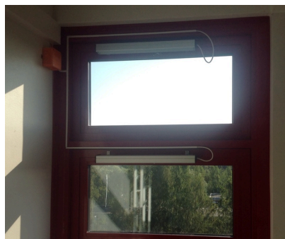
The smoke extraction windows of the staircase
