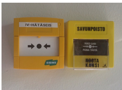
Air-conditioning emergency stop
