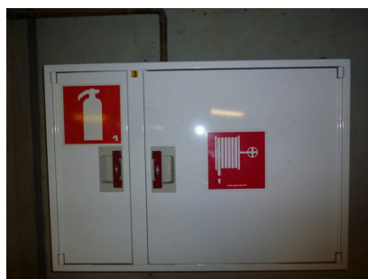
Initial extinguisher and fire hydrant
