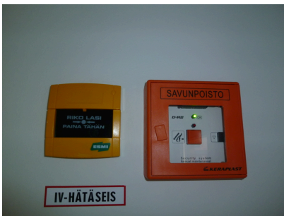
Manual smoke extraction activation
