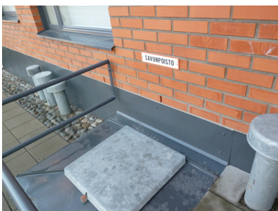
Smoke extraction hatch
