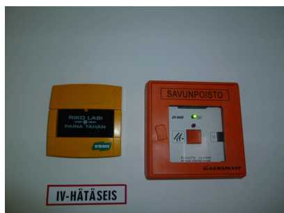
Air-conditioning emergency stop
