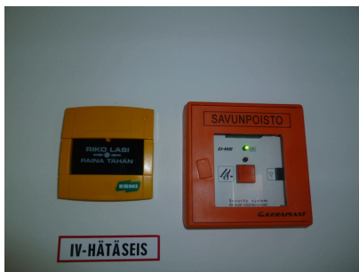
Air-conditioning emergency stop
