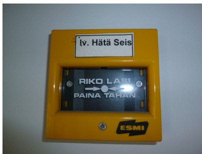
Air-conditioning emergency stop
