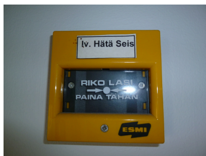
Air-conditioning emergency stop
