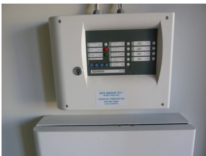
Fire alarm switchboard
