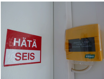
Air-conditioning emergency stop
