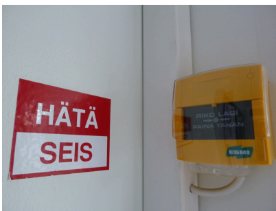
Air-conditioning emergency stop
