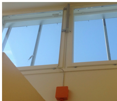
Smoke extraction window in the staircase
