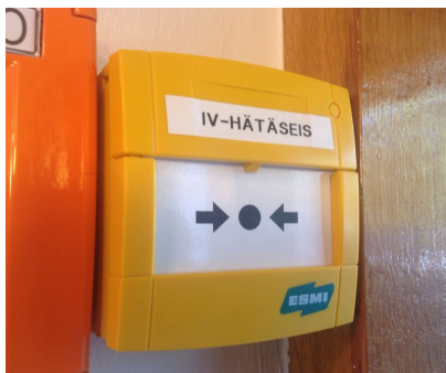
Air-conditioning emergency stop
