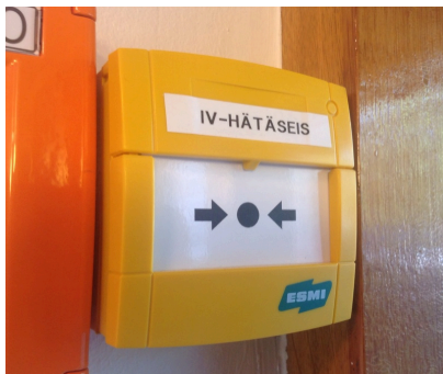
Air-conditioning emergency stop
